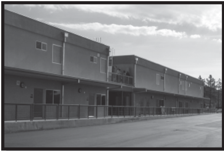
New Buildings at Hamilton School
