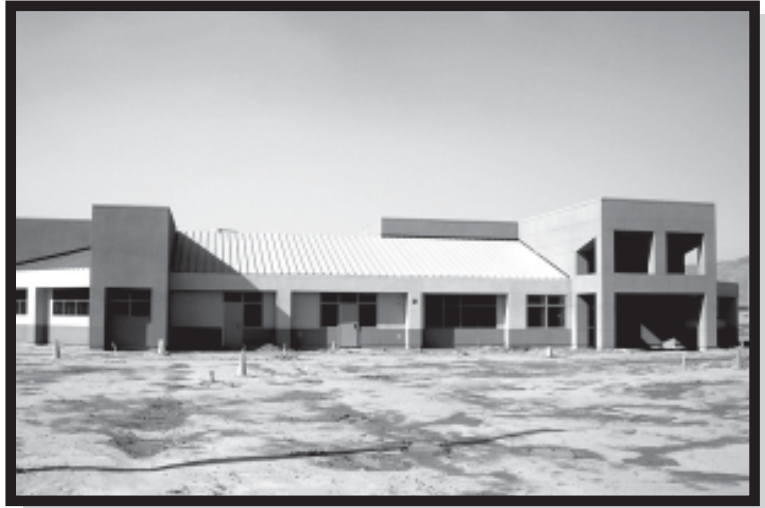
Tahquitz High School Construction Progress
